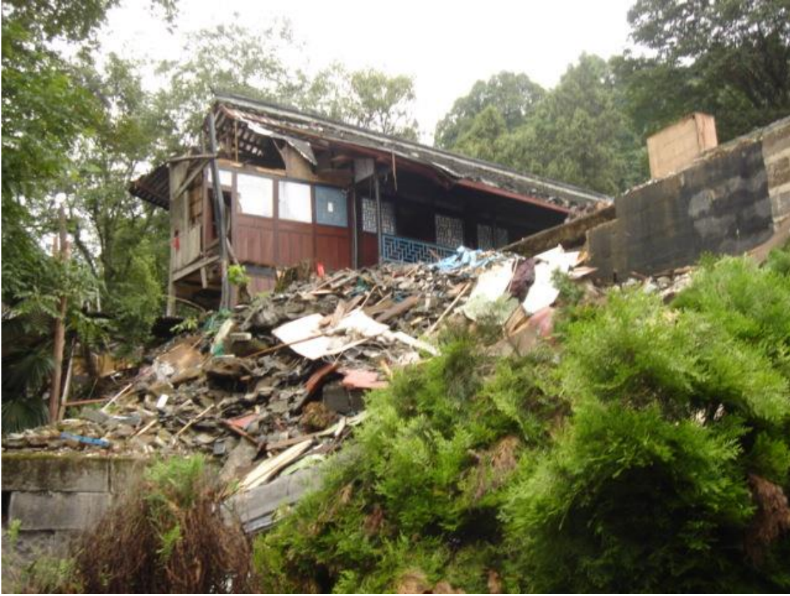
Figure 1.5. Earthquake Damage to a Local Historical Site in Dujiangyan (Source: Photo taken by Jia Lu, 2008)
