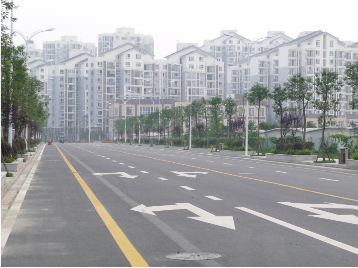
Figure 1.6. Post-earthquake Reconstructed Housing in Dujiangyan-01
