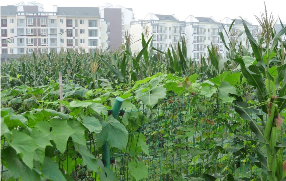
Figure 1.7. Post-earthquake Reconstructed Housing in Dujiangyan-02
