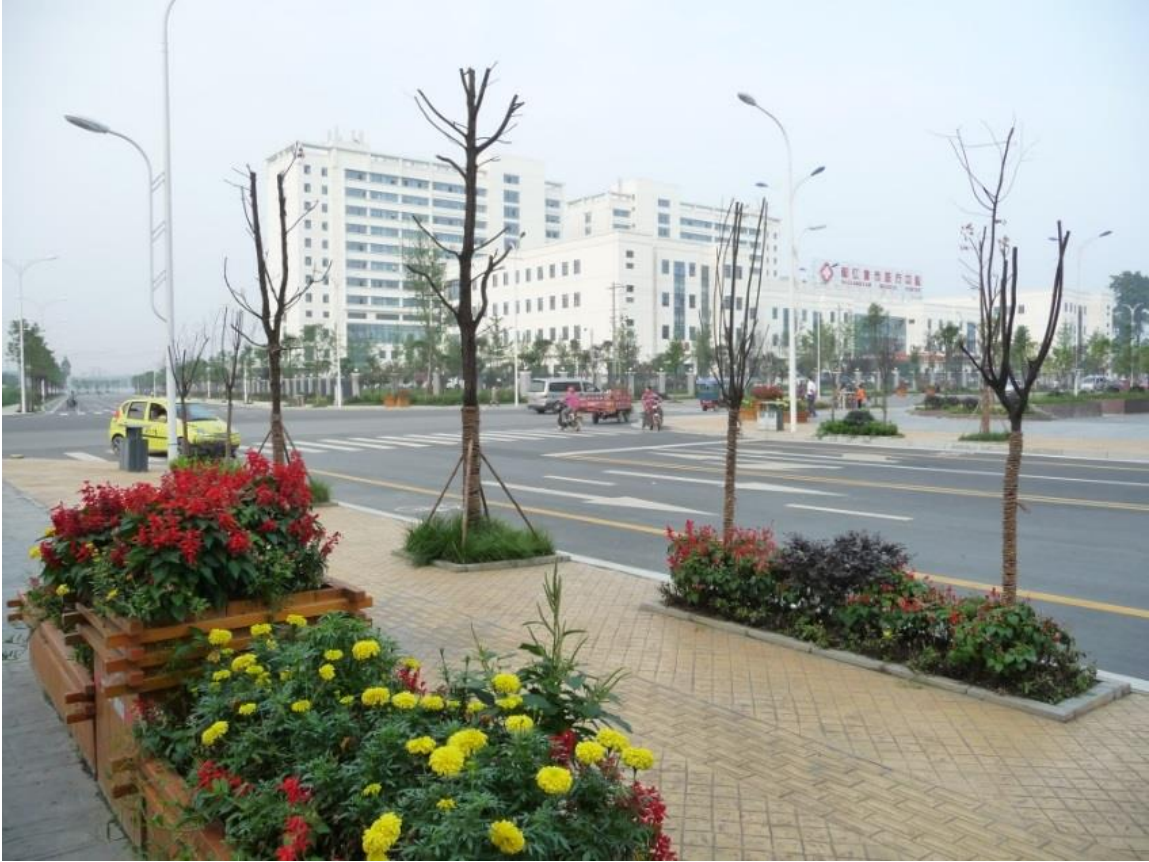
Figure 8.10.4. Newly Constructed Community Hospital Serving the Residents Living in Reconstructed Housing in the Surrounding Areas
