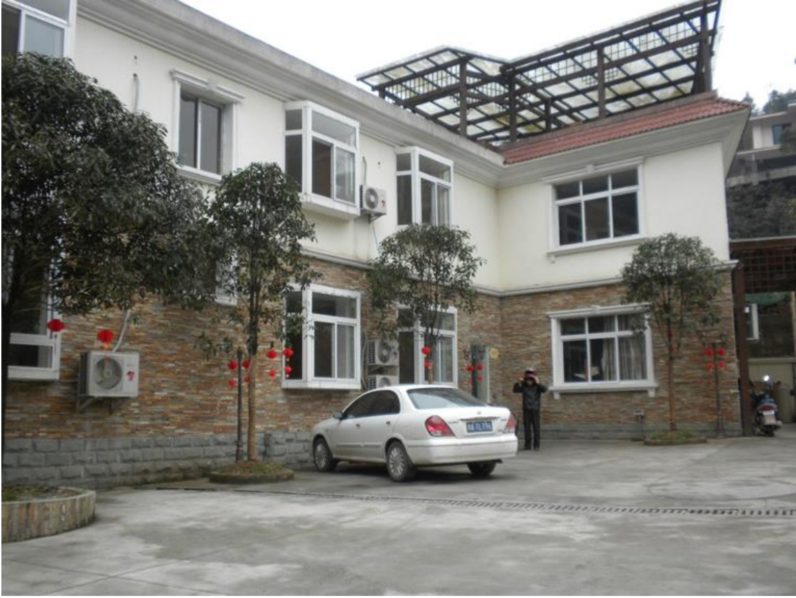
Figure A.3.8M. Chain Hotel Rooms Looking from Outside
